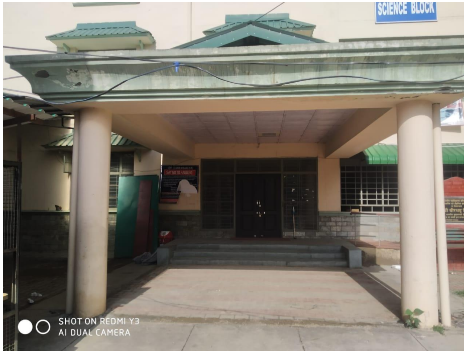
Fig:9 Proper Exit in Science Block
